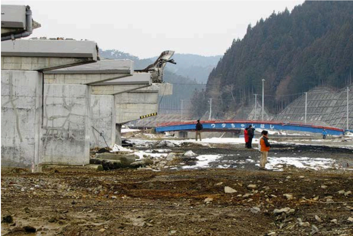
Figure 10 Bridge in Japan with complete wash out of the superstructure with only the piers remaining. Source: Structural Engineers Association of Washington.
