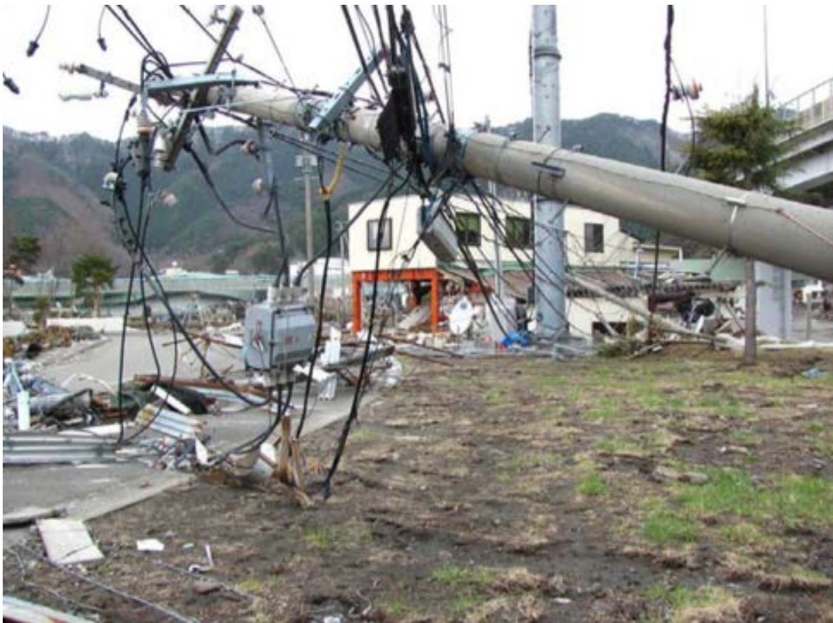
Figure 42 Damage to local electricity transmission lines from the 2011 Japan Tsunami. This would correspond to Damage State 1 in the analysis and Figure 43 below. (Source: TCLEE, 2010).
