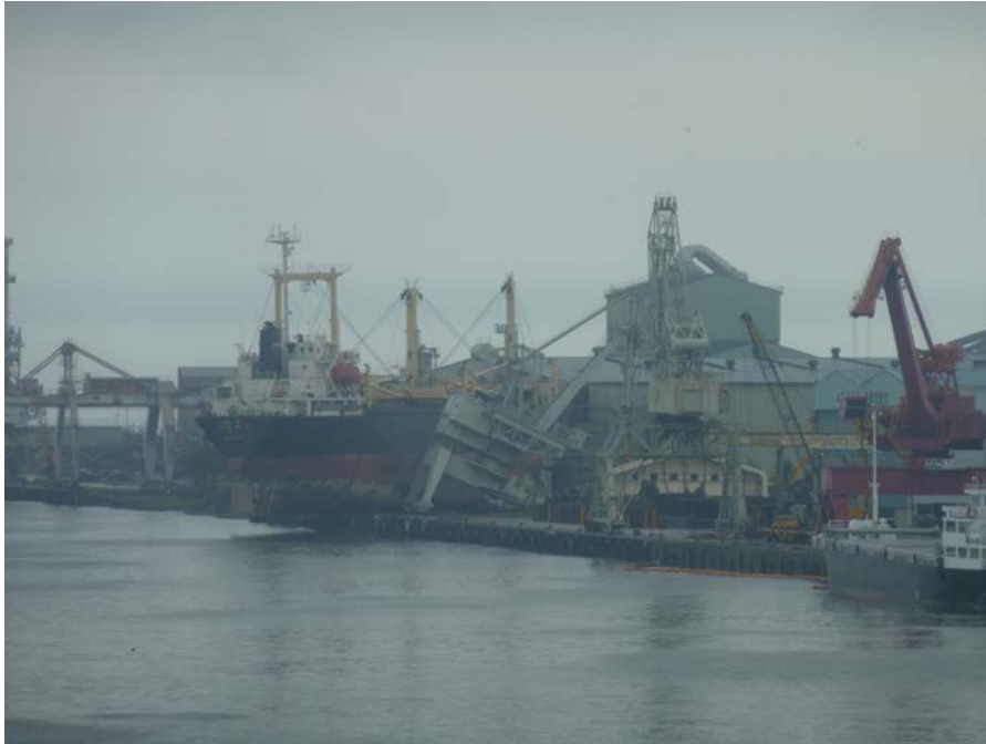
Figure 21 Example of damage to a gantry crane from debris strike by a large ship. Source: S. Fraser, 2011.
