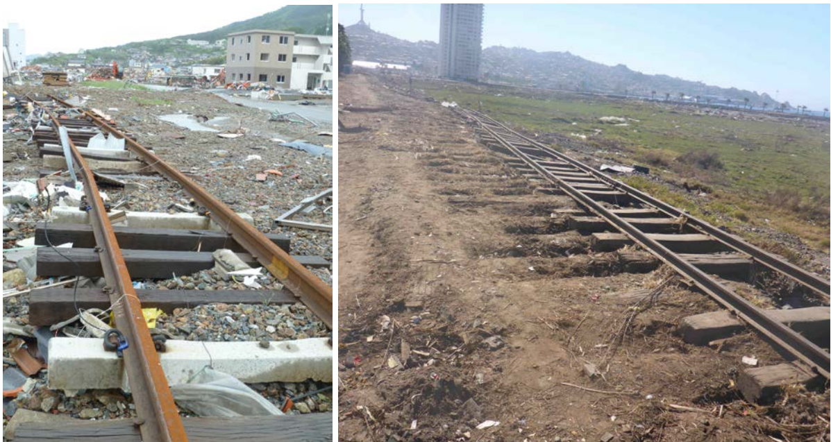
Figure 13 Scouring of rail ballast in Ofunato City, Japan, 2011 (Source: S. Fraser), and lateral movement and washout of a track in Coquimbo, Chile during the 2015 Tsunami (Horspool et al., 2016).
