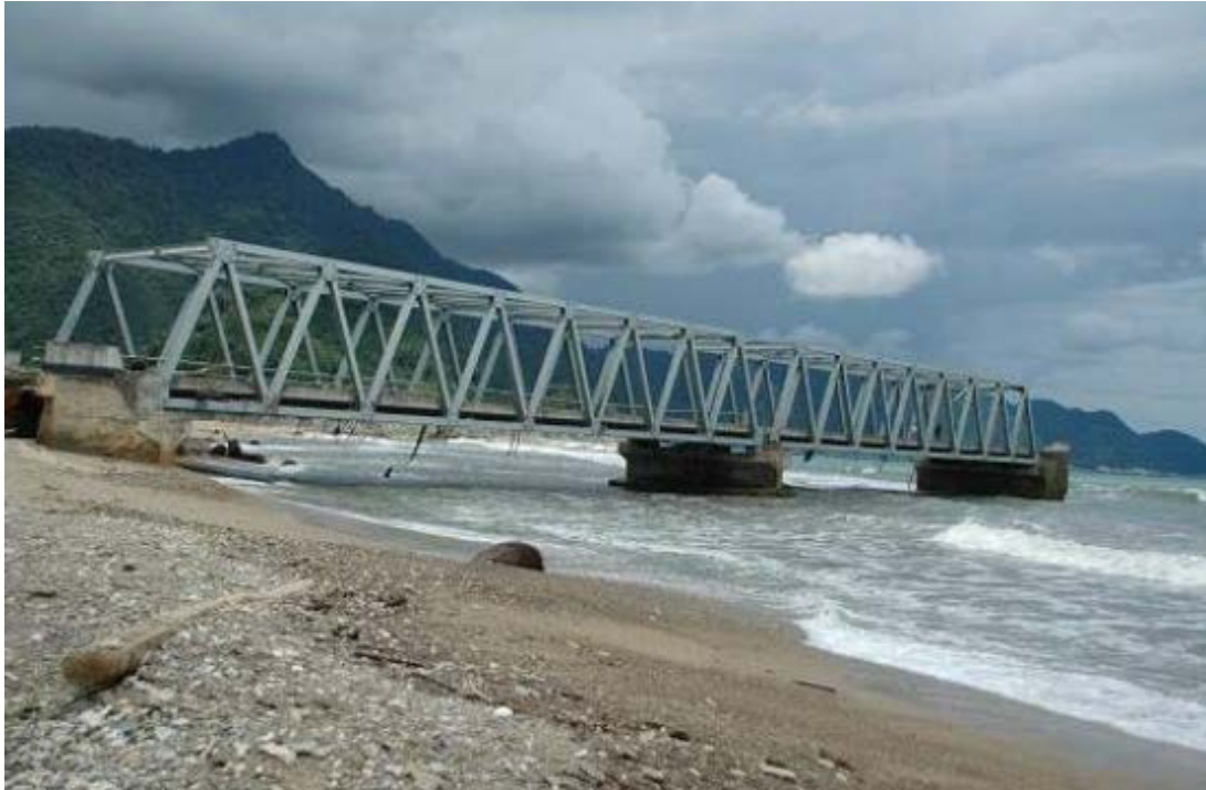
Figure 8 Bridge in Sumatra, Indonesia located on a river entrance, with complete scouring of one riverbank (right side of photo). Source: Francis, 2006.
