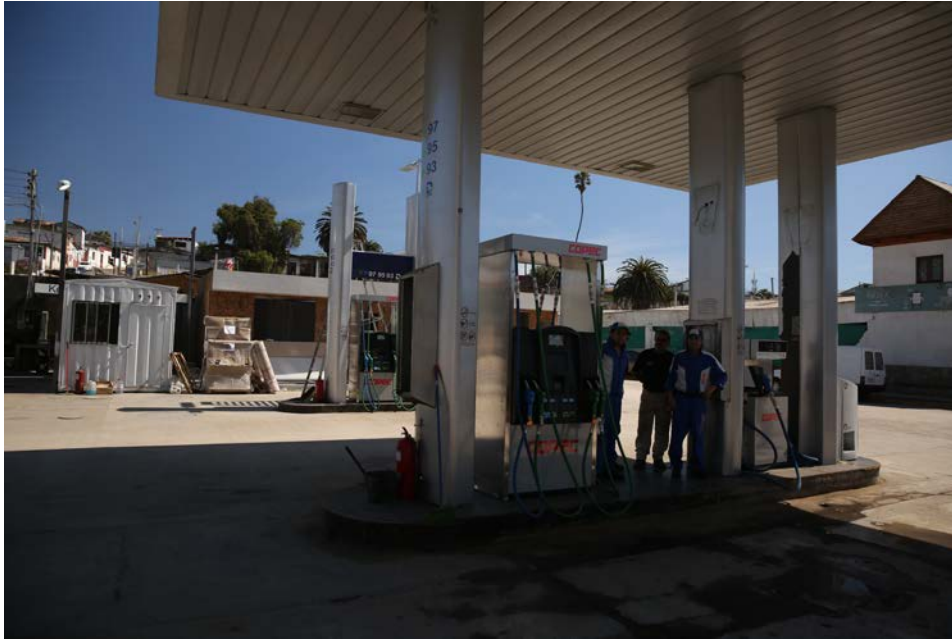
Figure 35 COPEC petrol station in Coquimbo, Chile damaged during the 2015 Chile tsunami. This photo taken 12 days after the tsunami shows the newly installed pumps and temporary retail building under construction (Horspool et al., 2016).
