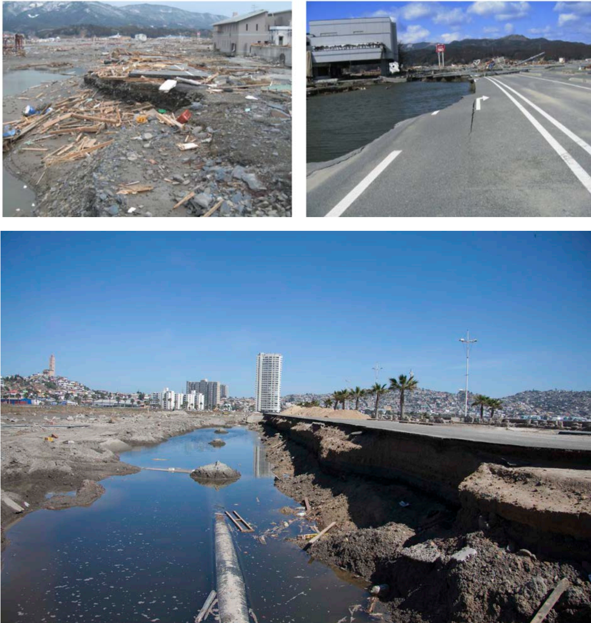
Figure 4 Upper Left: Peeling off of road surface in Iwate Prefecture (Unjoh, 2012), Upper Right: Scouring of road in Iwate Prefecture (Unjoh, 2012). Lower: Scouring of a raised coastal road and scour pit on the landward side of the road caused by the receding wave. (Horspool et al, 2016).
