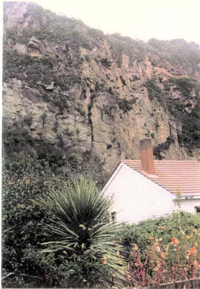
Rock face with obvious topple block. This type of column is very sensitive to outward rotation (Sumner area)
