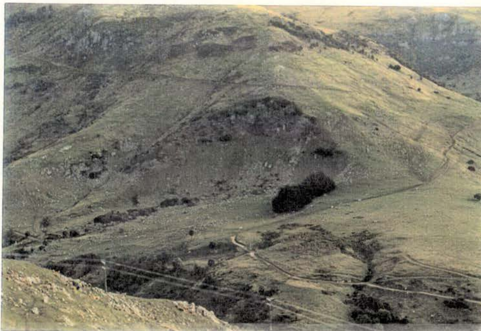
Old rock slide scarp. Failures on this scale are not common under static conditions and may have occurred during previous earthquakes
