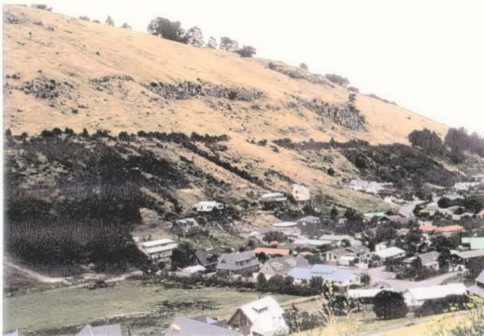
Steep slopes above housing with potential to generate significant damaging debris during an earthquake (Sumnervale Drive)
