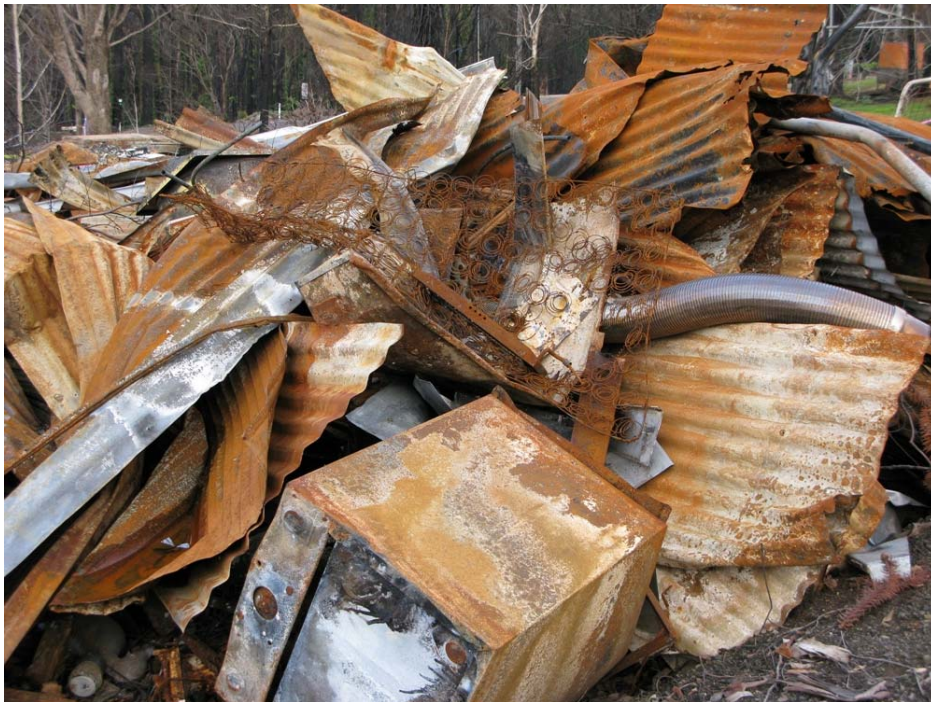
Figure 5 A pile of burnt metal ready for collection and recycling as part of the debris management programme following the Victoria Bushfires. The government appointed contractor elected to recycle metals and some vegetative and masonry items as part of their debris removal programme (photo Charlotte Brown).
