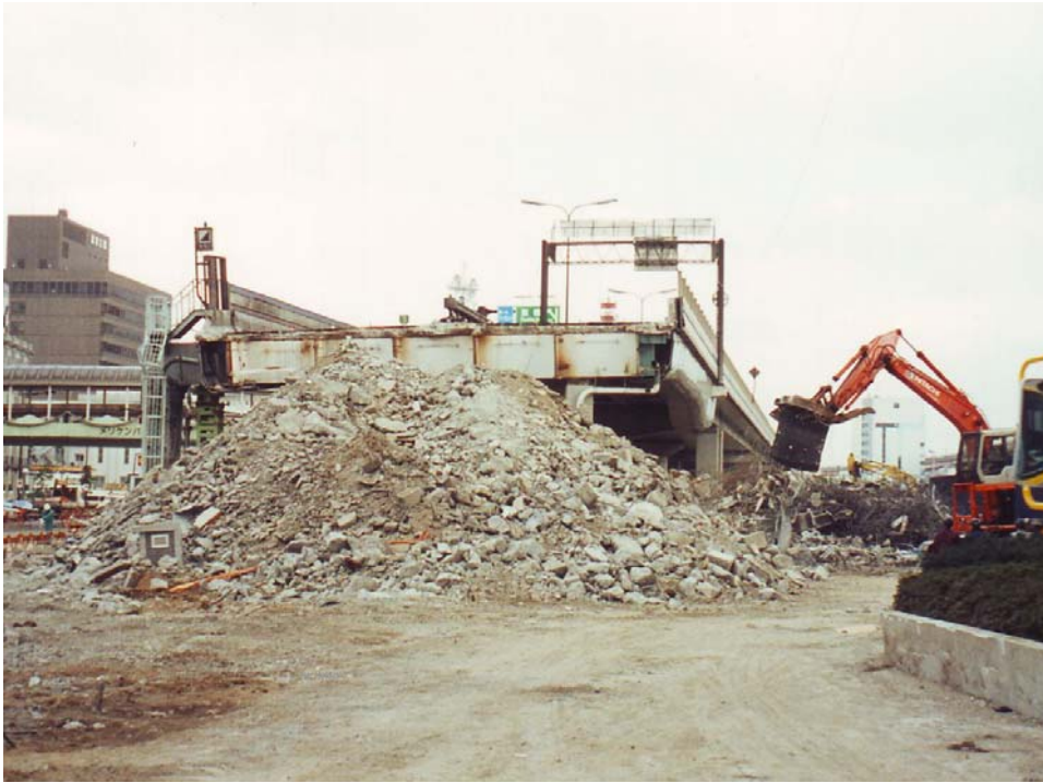
Figure 2 Remains of collapsed motorway, Kobe 1995 (photo Jim Cousins).
