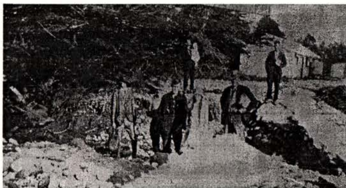
Figure 3-8. Quinlans Filling after the 1929 Earthquake - looking South towards Karamea (photo courtesy Karamea Museum)
