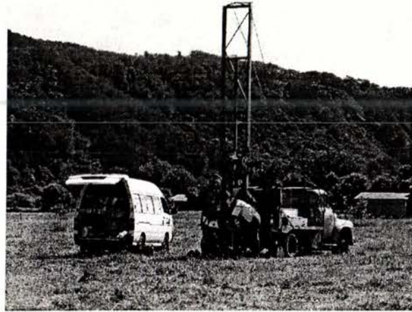
Figure 6-3. University of Canterbury Drilling Rig at Arapito (February 2003)
