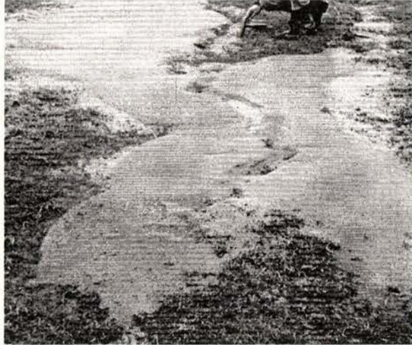
Figure 4-8. Sand Boils adjacent Hotham Street, Murchison (photo courtesy Dr. John Collen)
