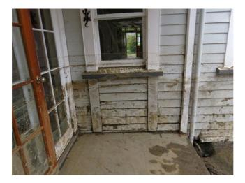
Figure 8 Moisture damage to weatherboards
