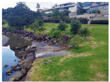
Figure 70 Riprap scour protection
