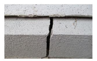
Figure 22 Cracked foundation
