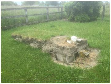
Figure 29 Displacement of septic tank
