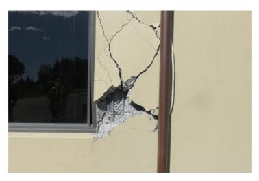
Figure 12 Cracked concrete panel
