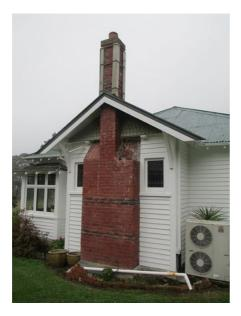
Figure 25 Chimney cracked at roofline with temporary supporting repairs
