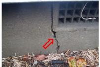
Figure 6: Old crack with paint embedment below East-facing window of dining area
