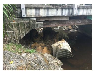
Figure 39 Impact damage to a bridge abutment from flood debris
