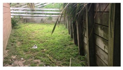
Figure 41 Timber retaining wall that has rotated due to land movement during a heavy rain event
