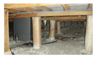
Figure 21 Pile detachment and rotation
