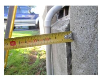
Figure 44 Out-of-plane displacement
