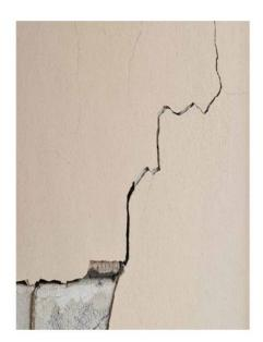
$\ \ Living\ room-1.5\ LM\ structural\ crack\ in\ painted\ plasterboard\ intertenancy\ wall.\ EQ-related.$
