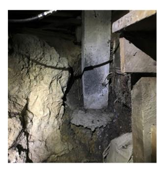
Figure 1 Pile settlement due to loss of support
