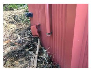
Figure 9 Impact damage to metal cladding
