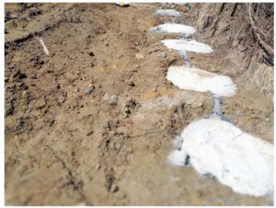
Figure 55 Reinforced concrete palisade wall – complete
