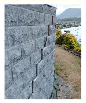
Figure 13 Step cracking to brick cladding with detachment
