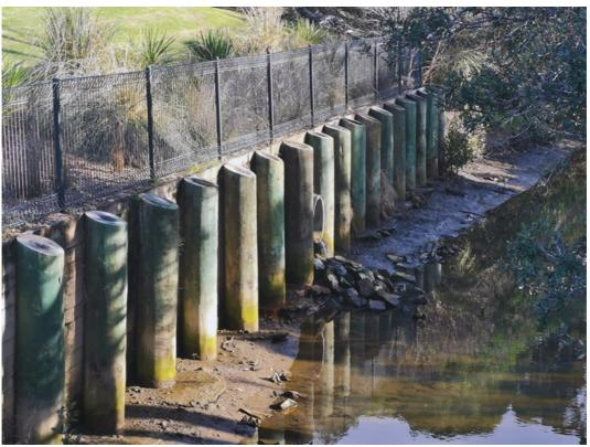
Figure 48 Timber pole retaining wall
