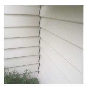
Figure 7 Weatherboard movement and cracking
