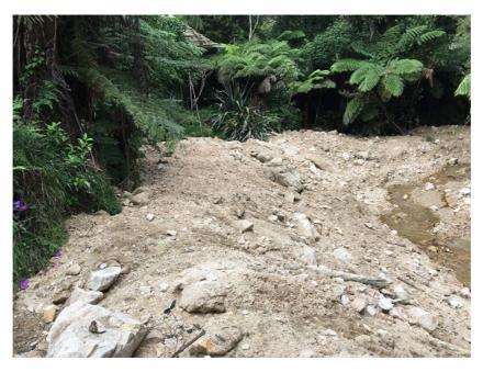
Figure 43 Stacked stone retaining wall washed away by flood waters
