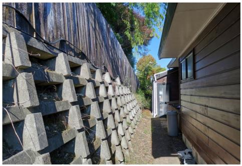
Figure 49 Concrete crib retaining wall
