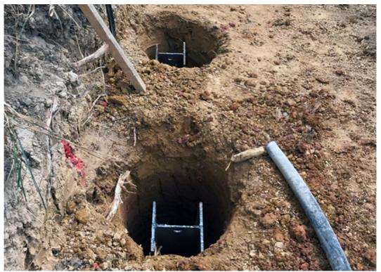
Figure 54 Reinforced concrete palisade wall holes
