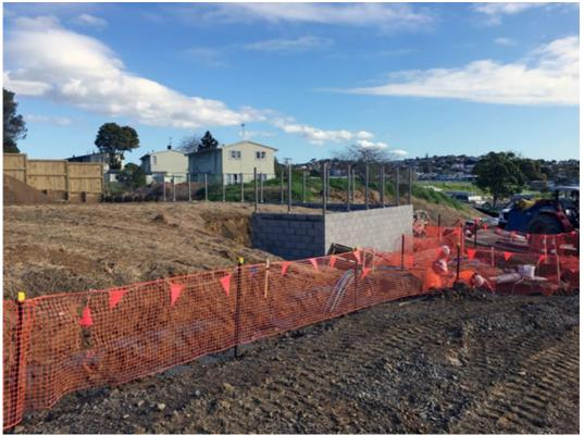
Figure 53 Concrete block retaining wall
