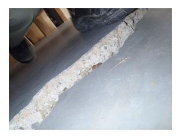
Figure 24 Cracking with vertical displacement
