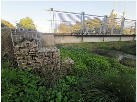
Figure 51 Gabion basket scour protection
