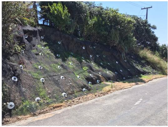
Figure 58 Soil nail retaining wall
