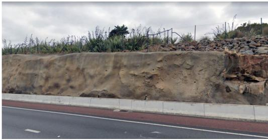
Figure 56 Sprayed concrete retaining wall
