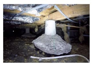
Figure 20 Loss of support resulting in settlement
