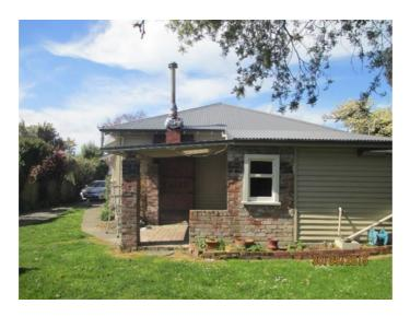
Figure 27 Disconnected flue with temporary waterproofing measures
