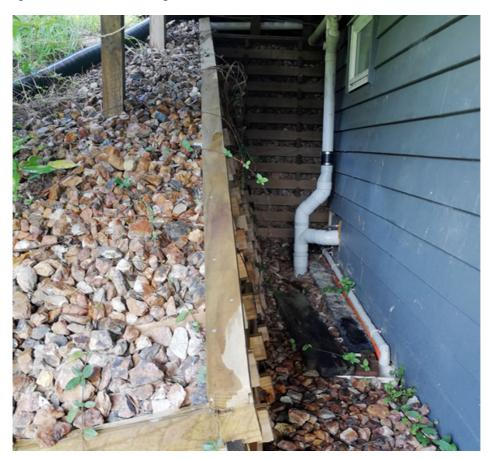
Figure 50 Timber crib retaining wall
