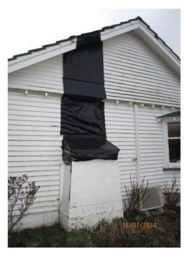
Figure 26 Total collapse of chimney with temporary waterproofing measures
