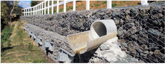
Figure 52 Gabion basket retaining wall
