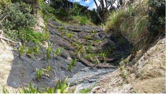
Figure 57 Pinned mesh retaining wall
