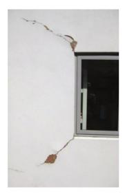
Figure 10 Cracked EIFS panel (BRANZ)
