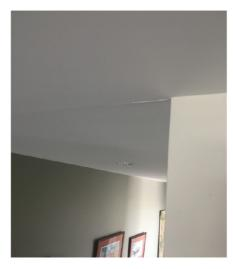
Hallway – 2.4 LM painted plastered ceiling crack. EQ-related
