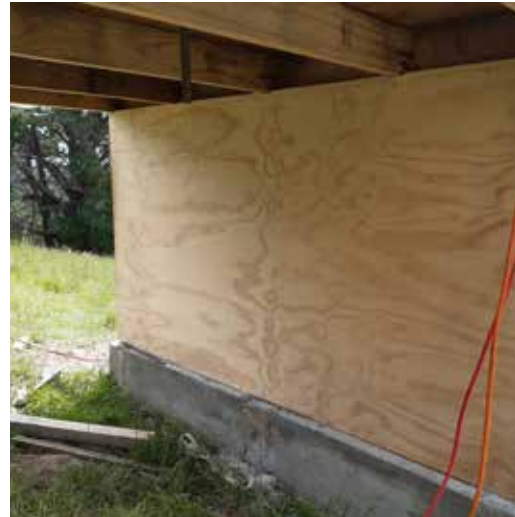
LEFT: ROGER SHELTON ON SITE FOR FOUNDATION TESTING. RIGHT: PLYWOOD DELIVERS EXTRA STRENGTH TO AT-RISK FOUNDATIONS.
