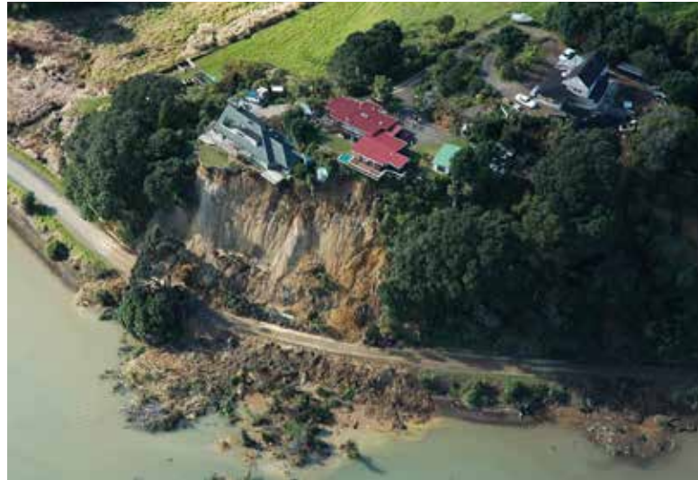
RAIN INDUCED LANDSLIDE, OHIWA, BAY OF PLENTY, JULY 2004 PHOTO CREDIT: GNS SCIENCE
