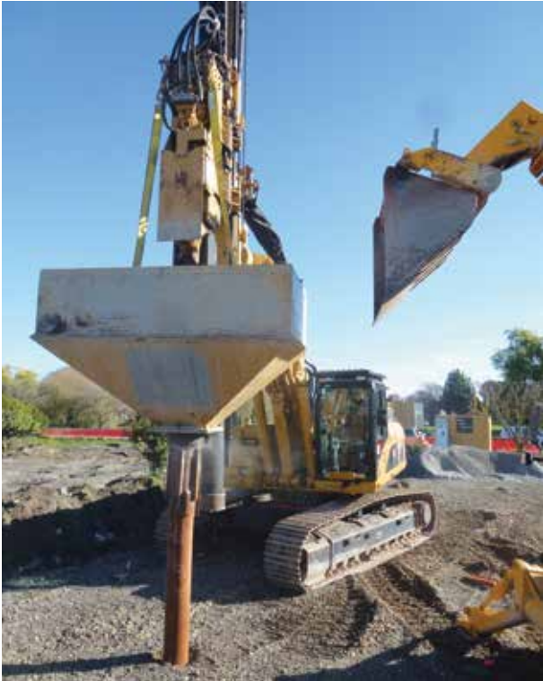
Equipment required to construct Rammed Aggregate Piers
