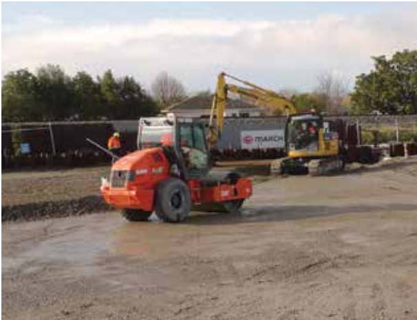
Roller compactor constructing reinforced gravel raft
