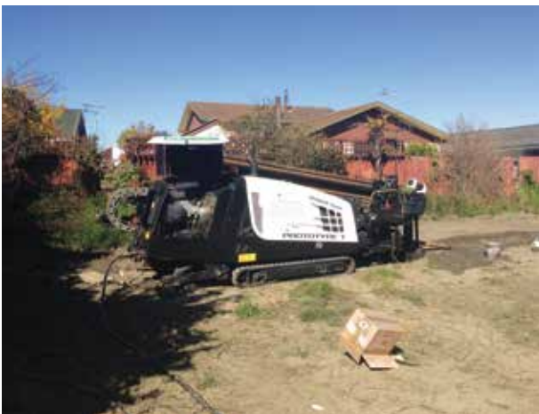
Directional drill constructing HSM beams
