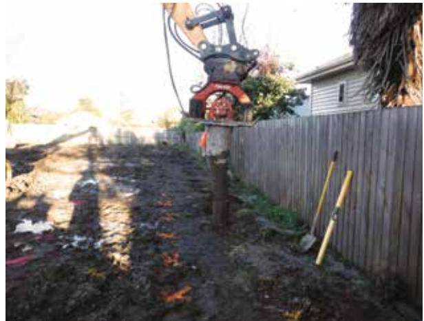
Construction of driven timber poles
