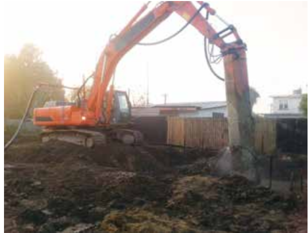
Construction of in-situ mixed soil-cement raft
