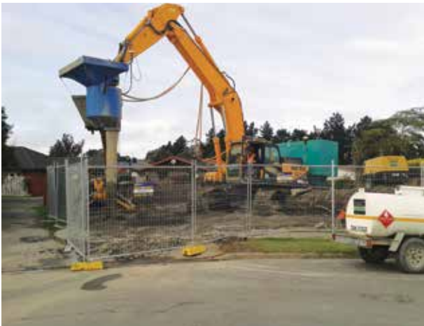
Construction of stone columns
