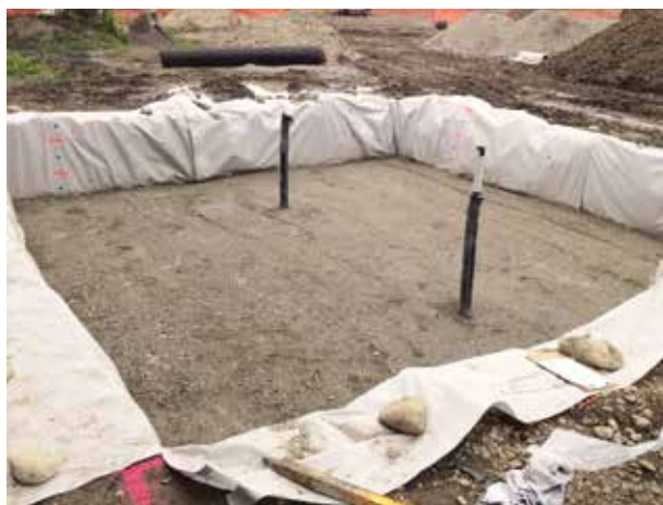
Construction of reinforced gravel raft test panel
