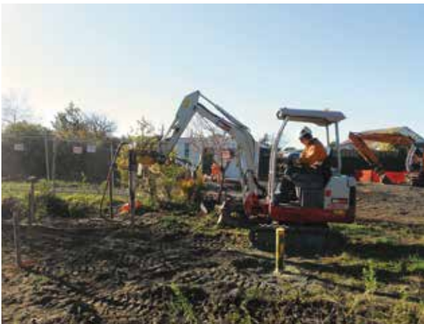
Installing steel casings for construction of low mobility grout ground improvement
