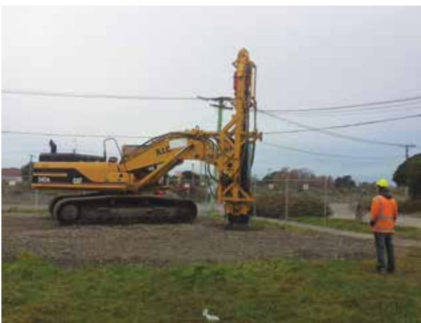
Rapid impact compaction equipment
