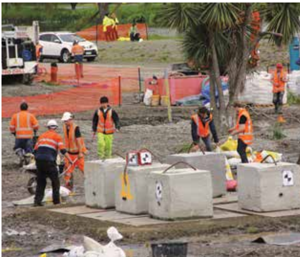
Preparation for blast induced liquefaction testing
