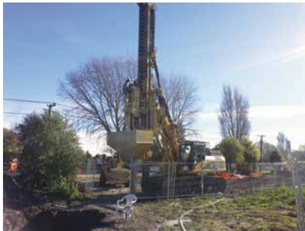
Construction of Rammed Aggregate Piers
